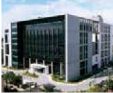
Taoyuan Technology Center (Green Building)
